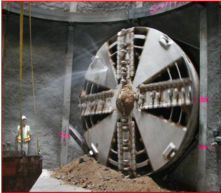
Photo of Tunnel Break-Through
