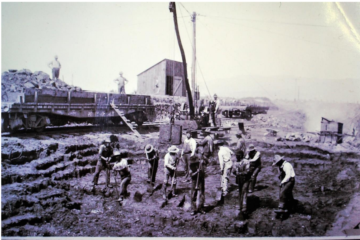
Figure 58. Alcatraz tar mine. Digging with hot shovels. Photo from Bob Gray.
