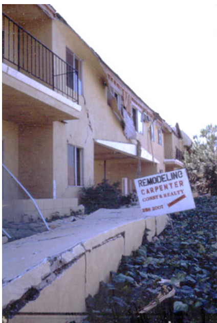
Photo 2. The scarp is just to the right of the photo and you can see the deformed sidewalk. Photo by Chris Reid. This close to the fault scarp, the hanging wall block was severely broken, with the convalescent hospital trashed and subsequently torn down. This exact location is now home to the I210-CA118 freeway interchange.
