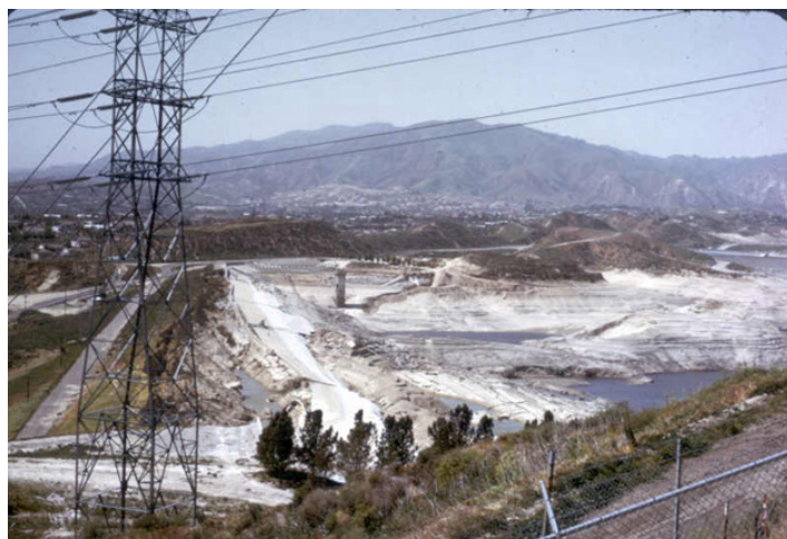
Photo 5. The Lower Van Norman Dam, looking west from the Odyssey Restaurant parking lot after the reservoir had been drained. The upstream face of the dam slid into the reservoir, taking out one of the two intake towers. The lake drained slowly, and at one point fire trucks were used to pump water out of the reservoir. Photo by Chris Reid. A smaller reservoir was rebuilt upstream a half mile upstream.
