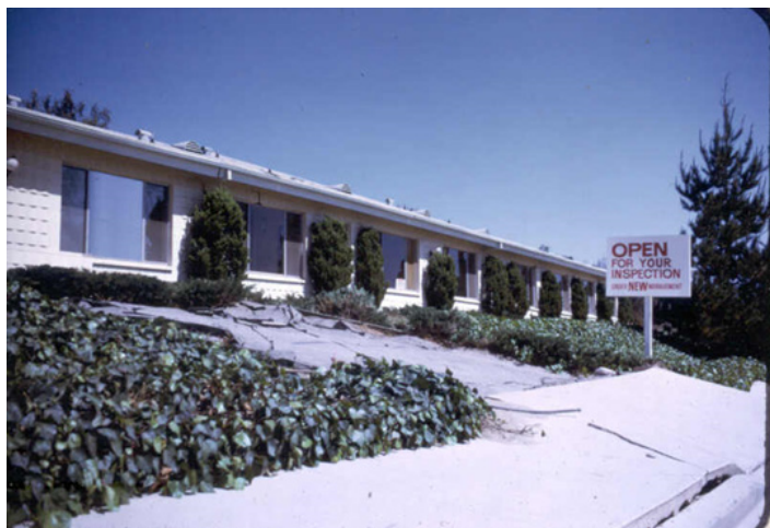
Photo 2. The scarp is just to the right of the photo and you can see the deformed sidewalk. Photo by Chris Reid. This close to the fault scarp, the hanging wall block was severely broken, with the convalescent hospital trashed and subsequently torn down. This exact location is now home to the I210-CA118 freeway interchange.
