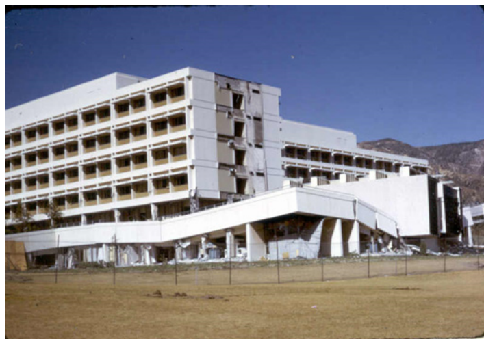
Photo 4. The recently completed Olive View hospital, located in an area of intense shaking on the hanging wall block. Note the collapsed stairwell structure and the damage to the second-floor columns. The structure was demolished and replaced with a new hospital. Photo by Chris Reid.
