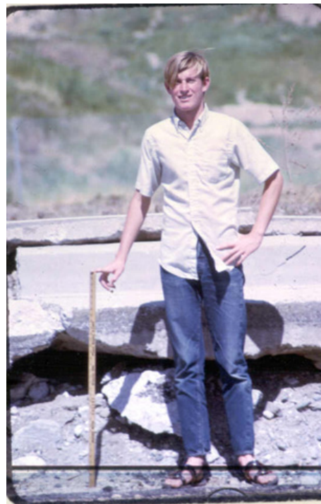
Photo 1. I'm standing on Foothill Blvd in Sylmar, holding a yard stick, in front of the fault scarp about a week after the earthquake. The curb and sidewalk behind me are uplifted about 3 feet. Photo by Chris Reid.
