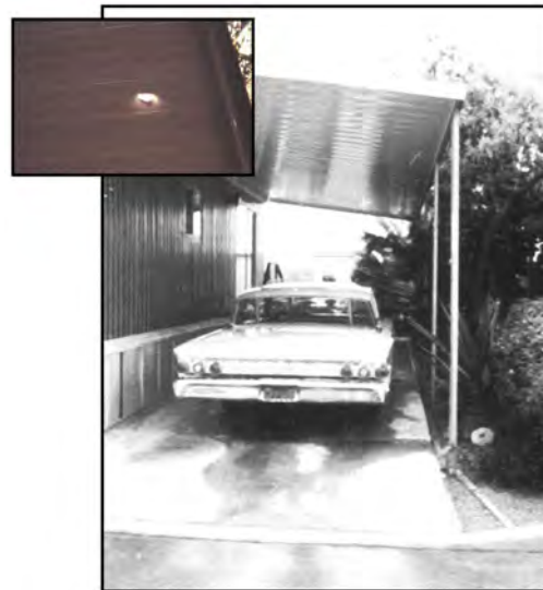
Figure 2: Jack Shurlock's aluminum carport roof at the Villa San Juan Trailer Park (now razed) that was struck by the San Juan Capistrano meteorite. Inset shows a close-up of the hole made by the stone; hole measured about 2" in diameter. The hole was located about 8" from the edge of the roof.
