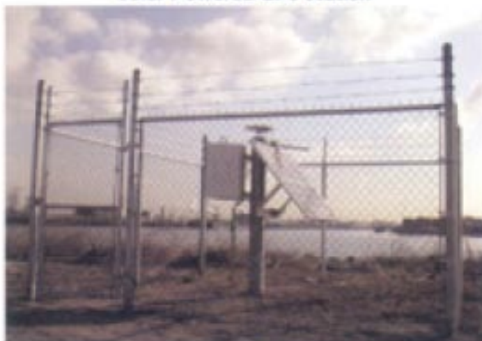
Solar Powered GPS Station
