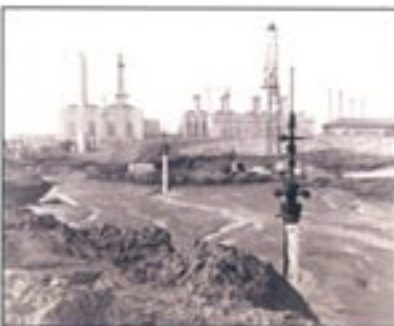
Well Heads Raised 20 Feet Prior to Adding Dirt Fill
