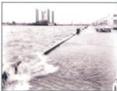
Wharf Awash in the Harbor Area at High Tide Due to Sinking from Subsidence
